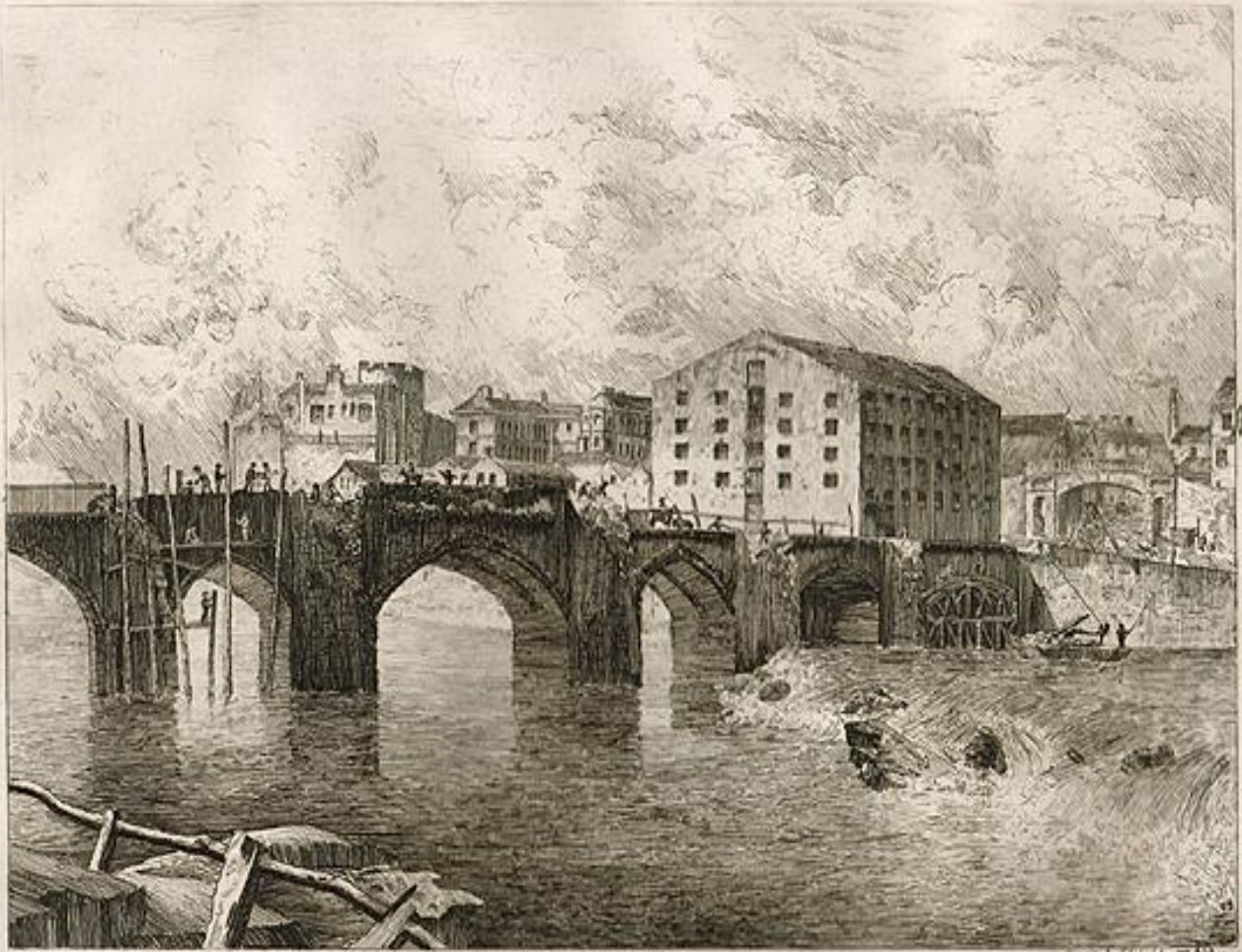
This year marks the bicentennial of the widening of the Old Dee Bridge in 1826. The bridge was widened by 7 ft. on the upstream side by adding an iron-plate footpath and railings, and the road surface was macadamized
