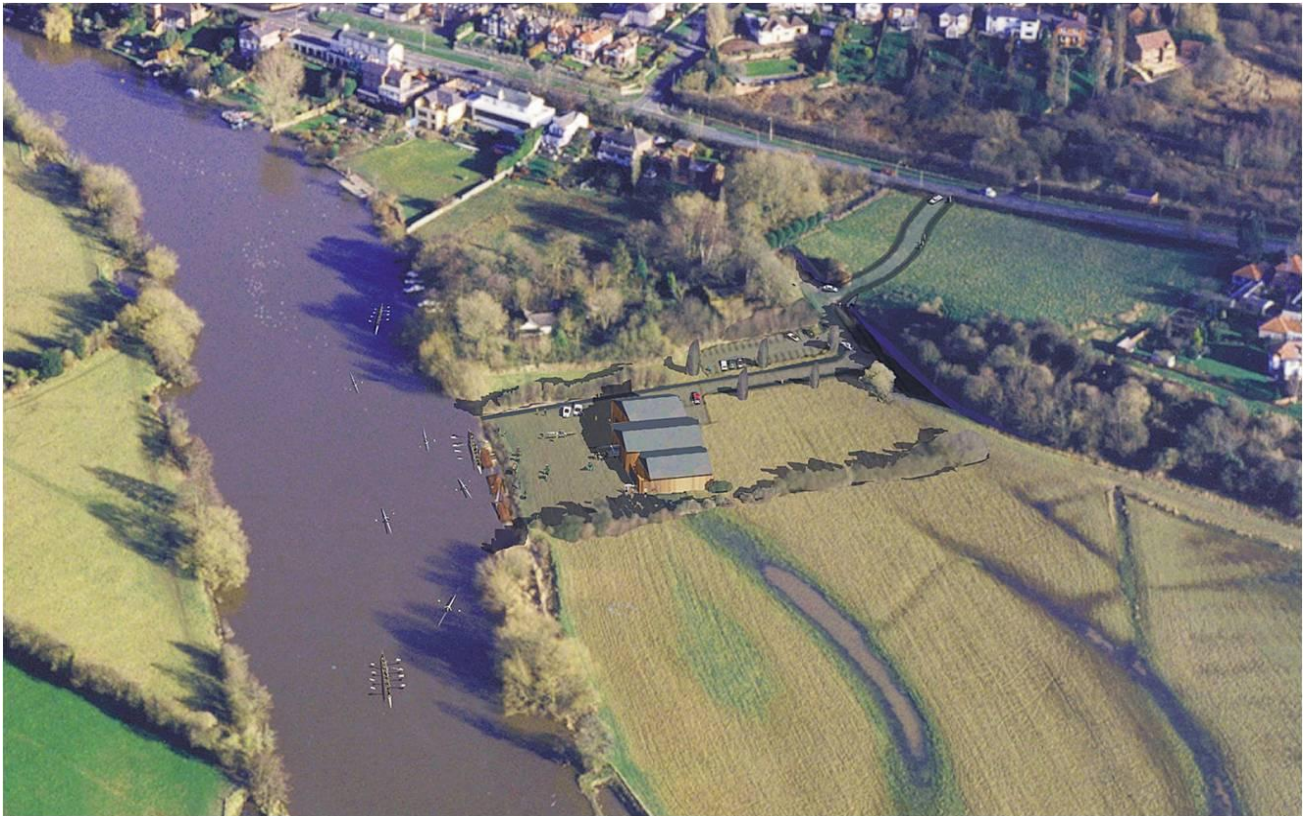
Aerial view of the proposed site
